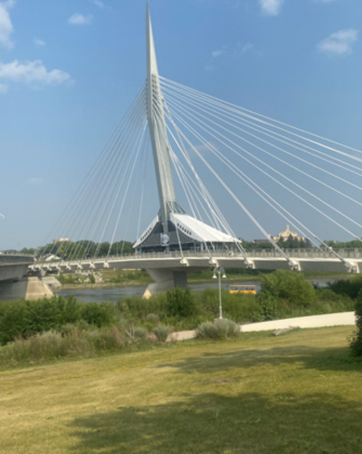
Esplanade Riel, a side-spar, cable-stayed pedestrian bridge that spans the Red River, is named after Louis Riel. Photo courtesy of Rebecca Chua
